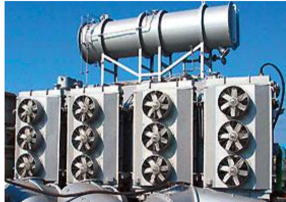
Transformer 400 MVA, EMS – TS Obrenovac
